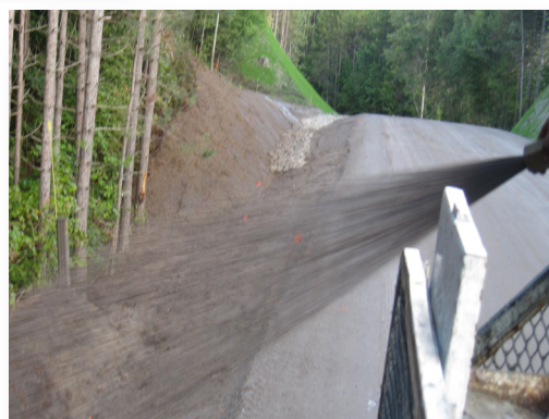
Top: Biotic Soil Amendment installation.
