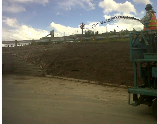
Biotic Earth is applied hydraulically, 2011.
