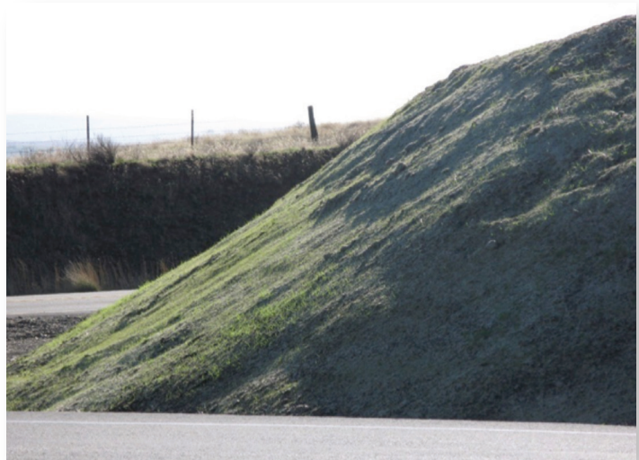
Results were evident immediately within the first year of installation.
