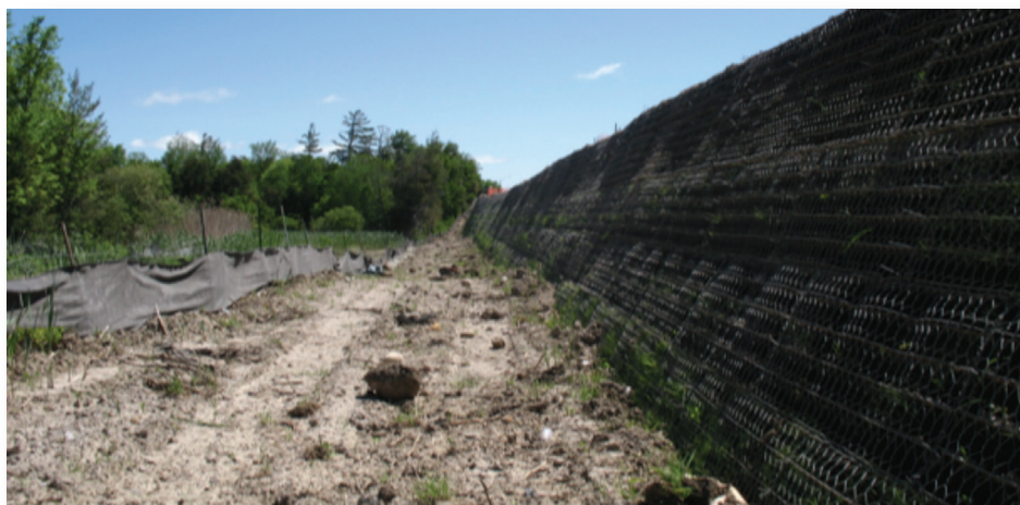
Early summer, 2010. Biotic Earth Black sprayed into Terramesh gabion green wall system.
