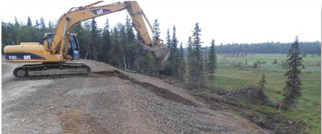
Importing topsoil was cost prohibitive on this project so vegetation was required on base material from the runway expansion.
