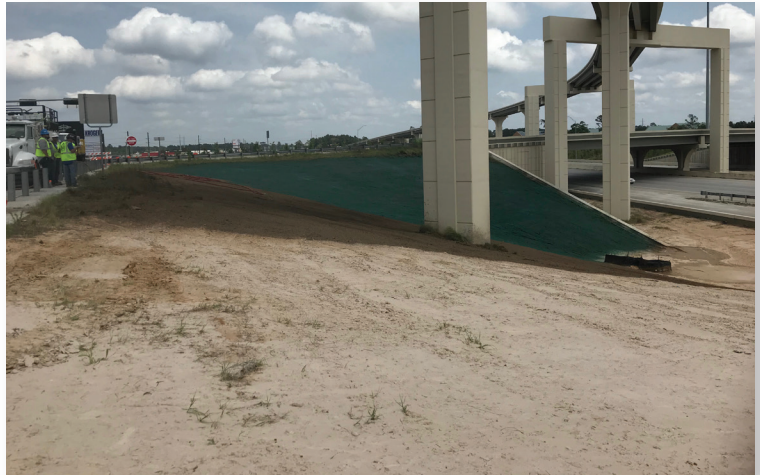
Applegate Woodlok HP covered the Biotic Earth for erosion control. March 2018.
