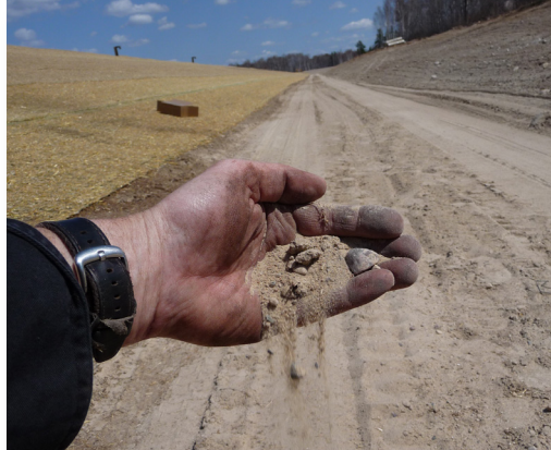
Existing soil on site was extremely sandy. Spring, 2009
