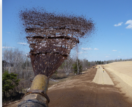
Biotic Earth is applied hydraulically. Spring, 2009
