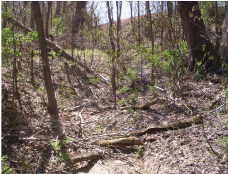
Previous attempts at using unreinforced vegetation had failed on the site.
