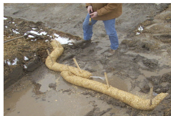
Overlap Sections 6 “ (min)
