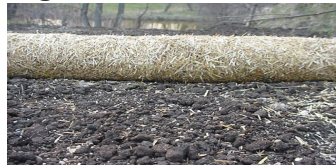
Good Stenlog/Soil Contact
