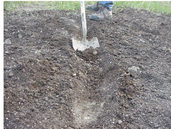
Dig Shallow Trench
